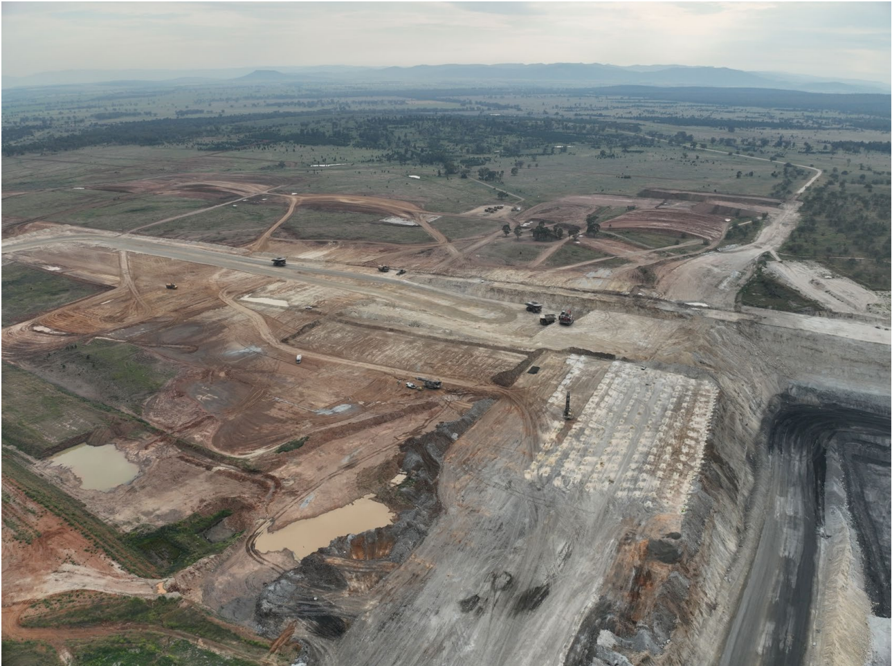
Figure 2: Image of recent clearing and soil stockpiles
