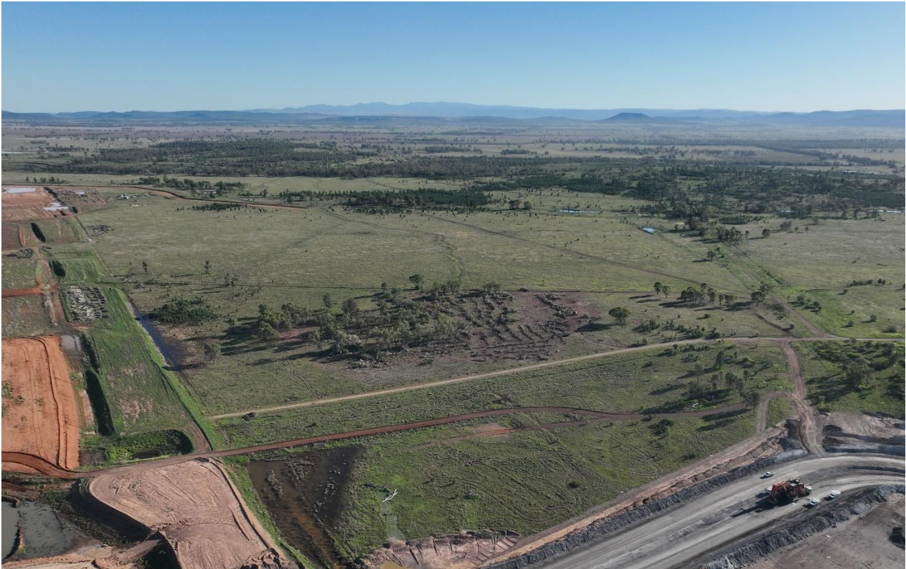
Figure 2: Image of recent clearing and soil stockpiles
