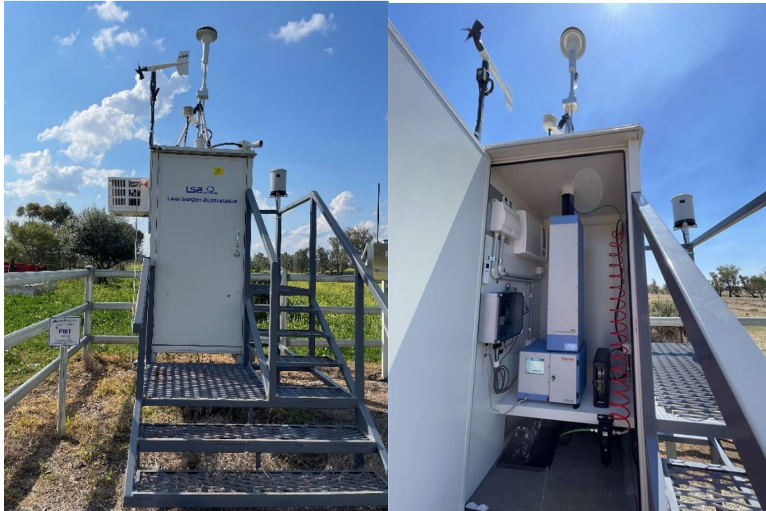
Figure 1: TEOM installed at Lanreef
