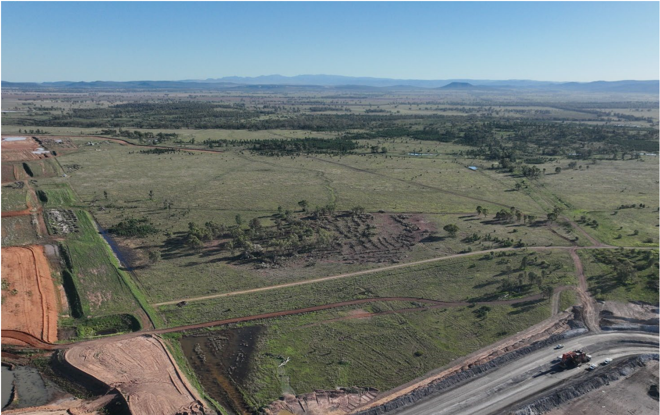
Figure 2: Image of recent clearing and soil stockpiles
